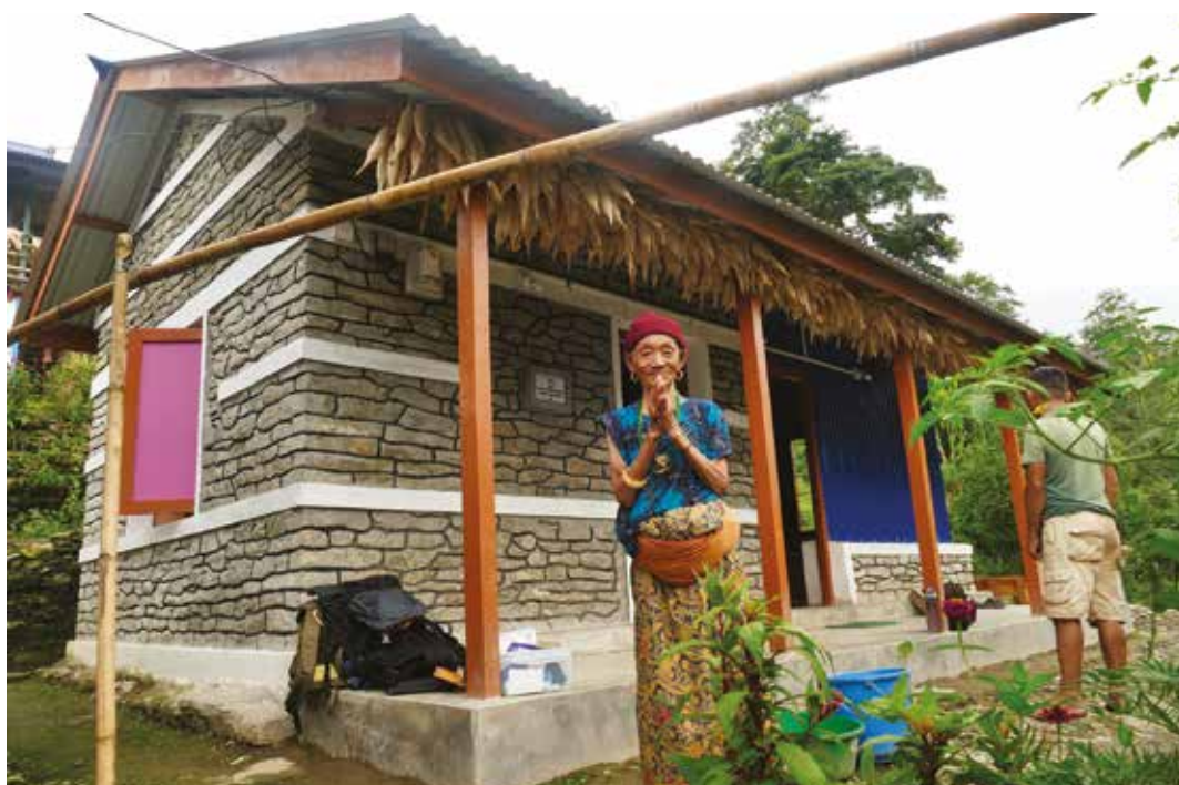
A GWT built earthquake-resilient home
