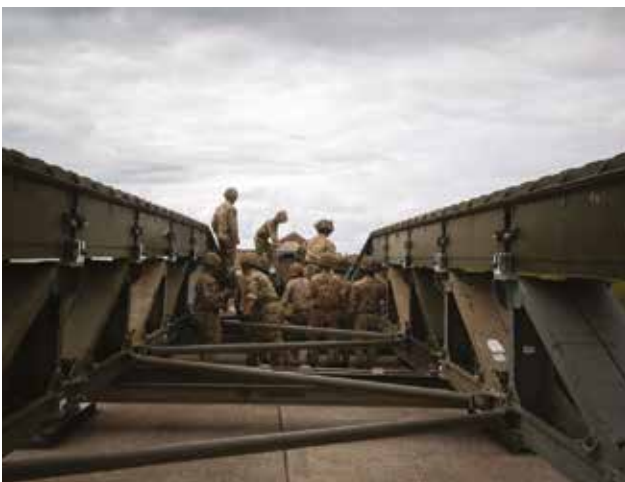
'Towards the gap', building a 12 Bay Double Story Medium Girder Bridge
