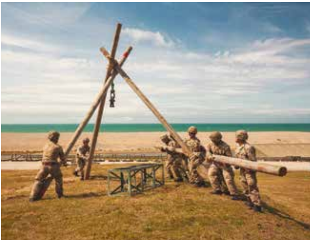
Sappers erecting an Aerial Ropeway, a skillset not often practiced
