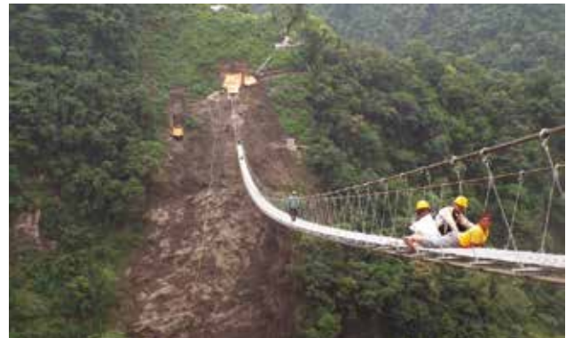
The bridge at Chomrong, spanning 287m
