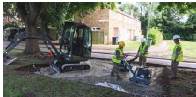
Sp Tp constructing Footpath at Invicta Park Barracks
