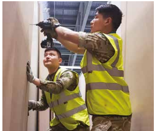
C & J constructing the ICU cubicles
