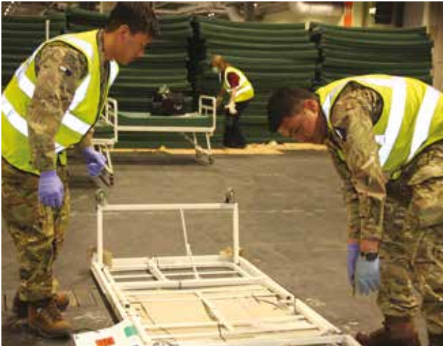
248 Gurkha Signal Squadron deployed to assist in the construction of the emergency Covid hospital in Birmingham
