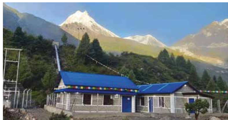
Sama Gaon hydroelectricity plant
