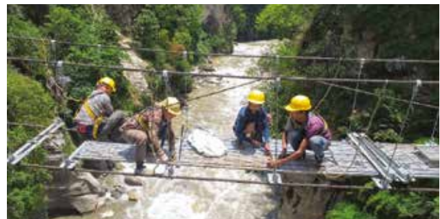
Decking out a suspension bridge
