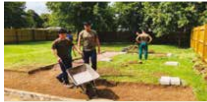
94 Sqn personnel constructing the messing hut area
