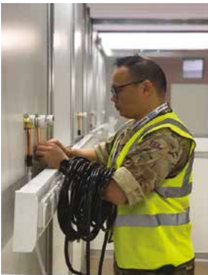
H&P installing medical gas hoses
