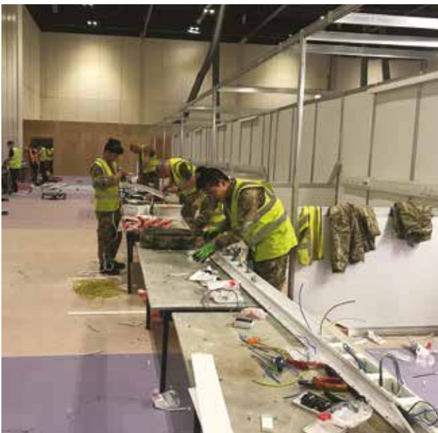
QGE - providing a helping hand in building NHS NIGHTINGALE London
