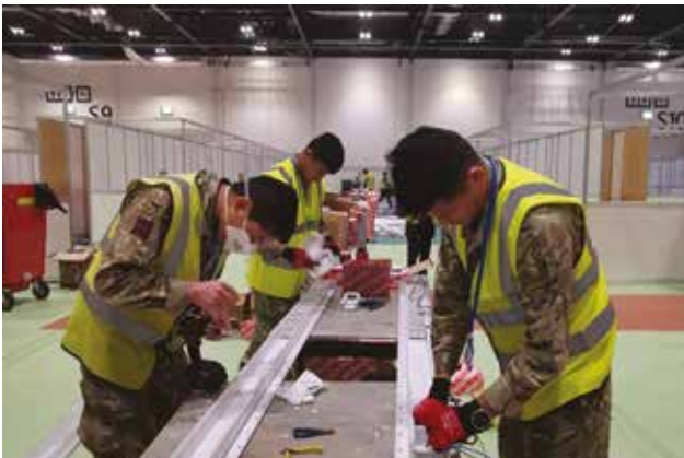
Military and Civilian Electricians preparing trunkings for ICU cubicles
