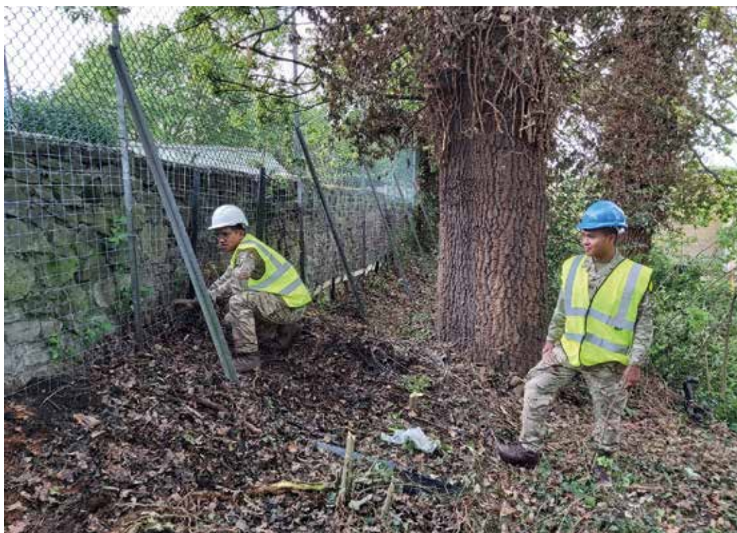
Cpl Gyanendra inspecting the fence upgrade work
