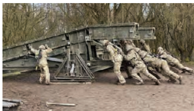
Construction of 12 Bay MGB DS during Ex INVICTA STALLION
