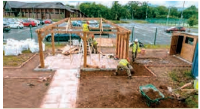
Brecon High School Project - Construction Phase
