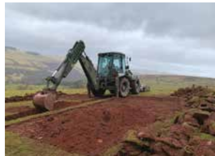
Defensive harbour construction
