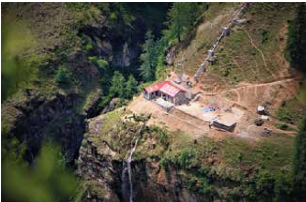
Chumling micro hydroelectric plant in NE Gorkha
