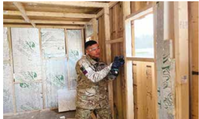
Spr Subash on FOB Upgrade Project
