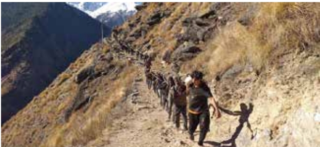
Villagers carrying a bridge cable
