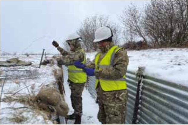
IBS Brecon - Pic 3. IBS 03 Russian trench refurbishment
