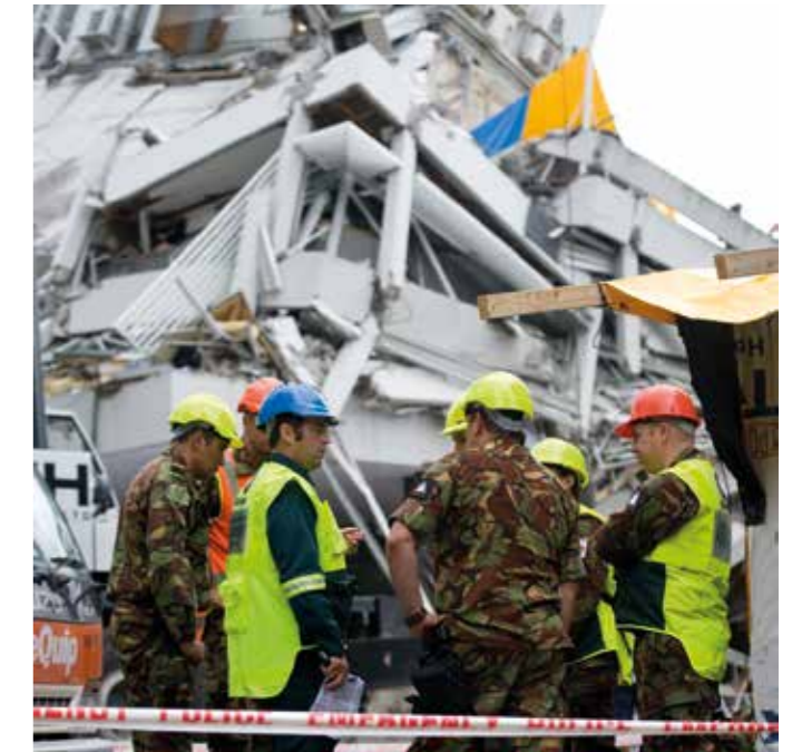
The Army and USAR discuss the ongoing rescue from collapsed buildings in the central business district of Christchurch.
